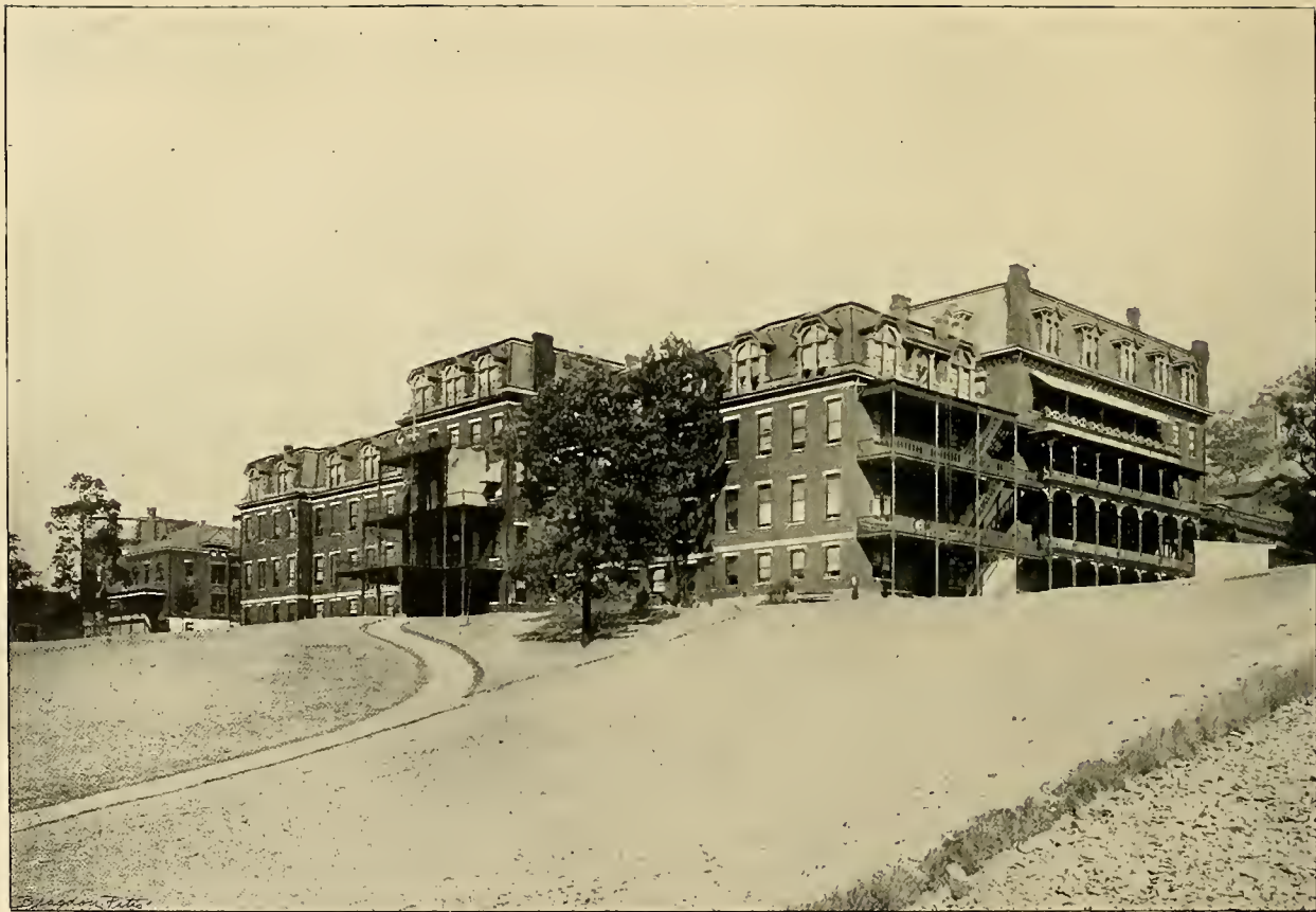
Western Pennsylvania Hospital, Twenty-eighth Street and Pennsylvania Railroad.
